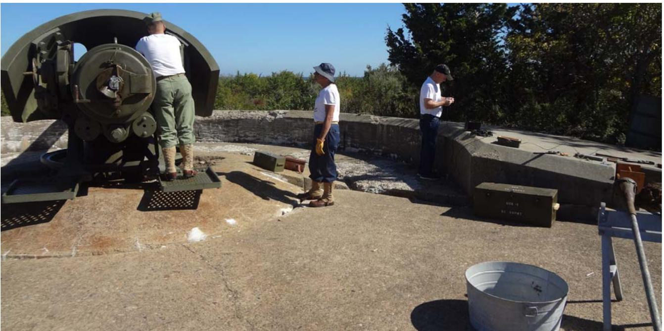
Here, T-5 Richard King installs a c. 1915 platform light for Gun No. 1. This is one of only four such lights restored in the nation, all of which are at Battery Gunnison/ New Peck. He and T-5 Komorowski developed a new method for safely and efficiently mounting the platform lights this past fall.
